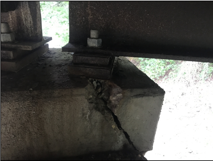
Bent 3 span 3 pillar block bearing pad has large delamination under bearing
