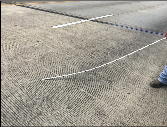
Transverse and longitudinal cracks in span 1 of the deck.
