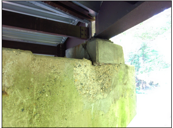
Bent 3, span 3, girder 1: pedestal is cracked and delamed under the bearing. Approximately half of the bearing area is compromised. 2022
