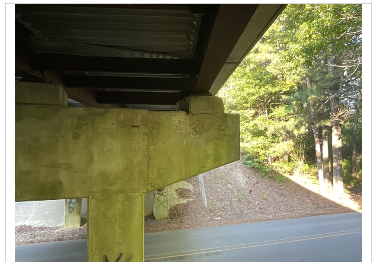
Bent 3, girder 1: cap is spalled.
