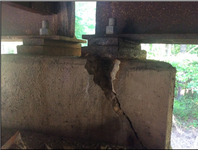
Bent 3 girder 1 raised bearing seat has a spall under bearing, also a crack that extends through the riser under the bearing.
