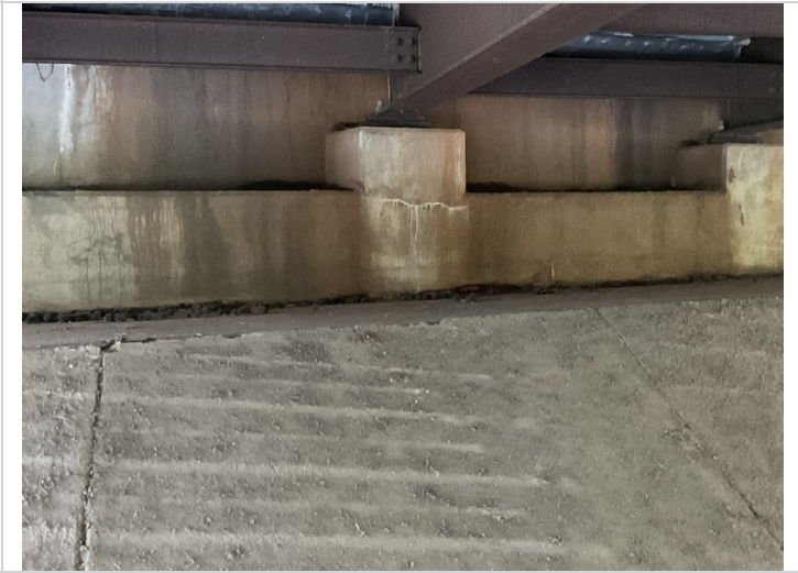
Bent1, girder 4: pedestal has transverse crack with efflorescence staining. Similar condition at bent 4, pedestals 4&5.
